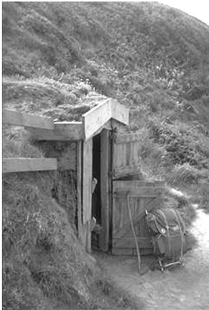
Hawker's Hut was built by the Reverend Robert Stephen Hawker who was the vicar of nearby Morwenstow church for 40 years from 1834. It is constructed of drift-wood collected from along the coast and nestles into the hillside. It is now in the care and protection of the National Trust and it is probably their smallest property! The vicar was responsible for giving a Christian burial to sailors who were drowned in wrecks along the coast and he used the hut to watch for wrecks and to write poetry.
