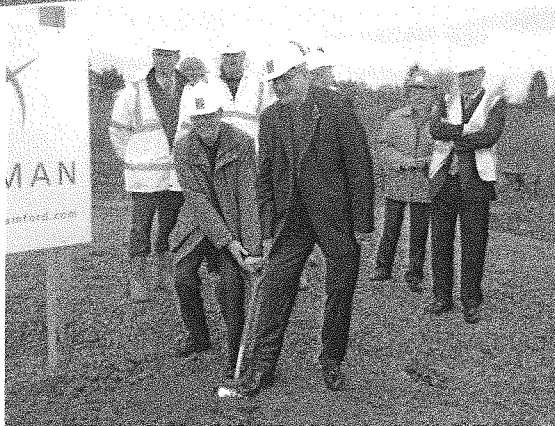
Photos: Bishop Stephen breaking ground at Stanground with Stephen Betson, Canon Malcolm Griffiths, David Hicks and representatives of the local council and the contractors
